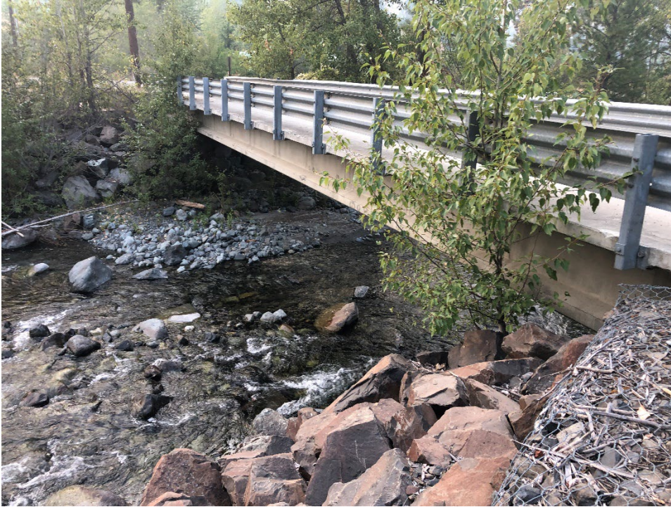
Figure 11. Private bridge over Peshastin Creek near Highway 97.
