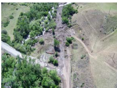
Aerial Shot of Flooding
