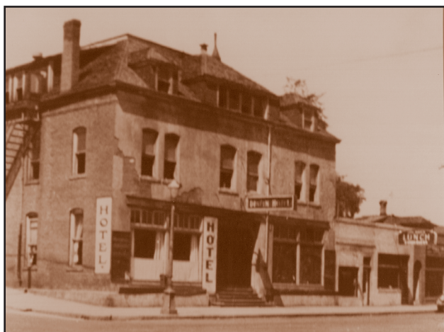
The county sold the courthouse to John Doneen, who operated it as a hotel for about 15 years.
