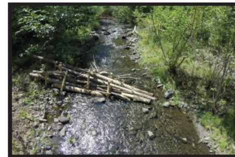
Figure 37. Typical structure schematic for a bank-attached post assisted log structure used to force a constriction jet.
