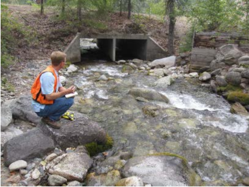
Photo 1: Upstream of the Twenty-Five Mile Creek culvert.
