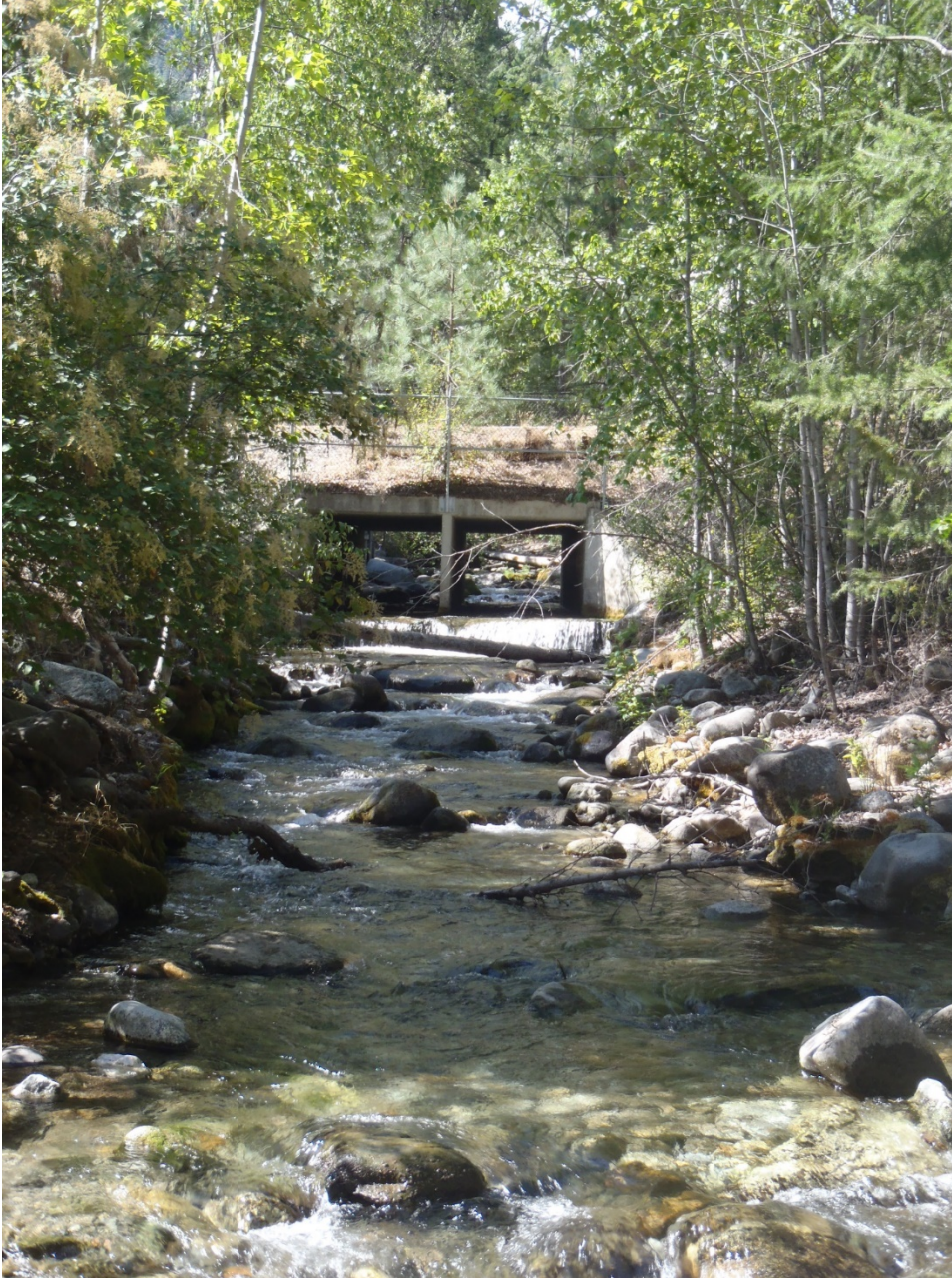
Photo 3: Downstream of the Twenty-Five Mile Creek culvert.
