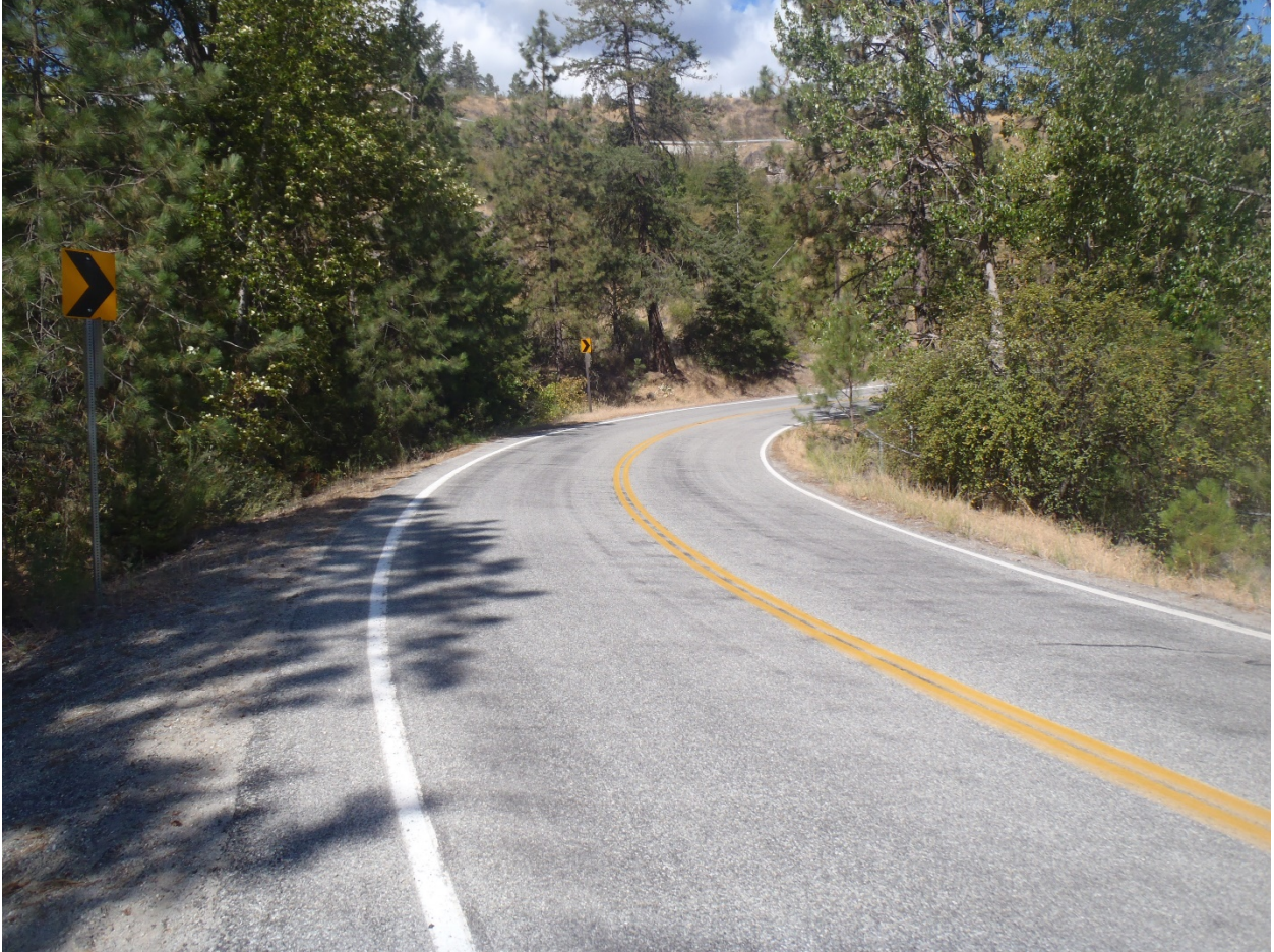
Photo 5: Looking West towards the culvert along South Lakeshore Road.
