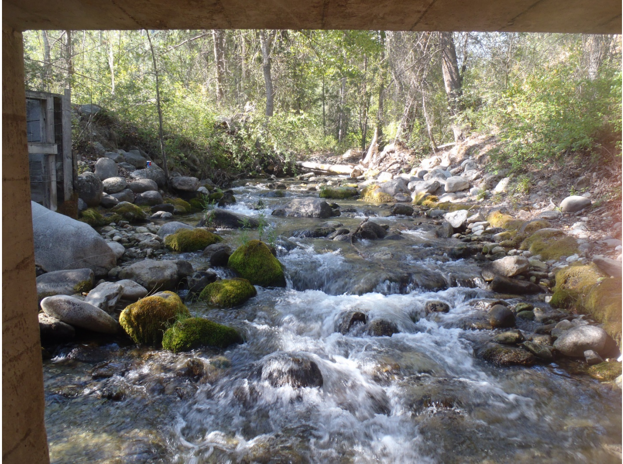
Photo 4: Upstream of the Twenty-Five Mile Creek culvert.
