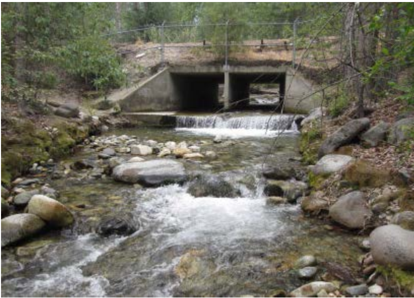
Photo 2: Downstream of the Twenty-Five Mile Creek culvert.
