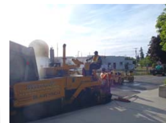
(Left) Paving the Mainline on Wapato Way
