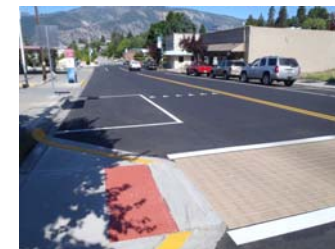
(Left) Upgrading ADA Ramps & Crosswalk
